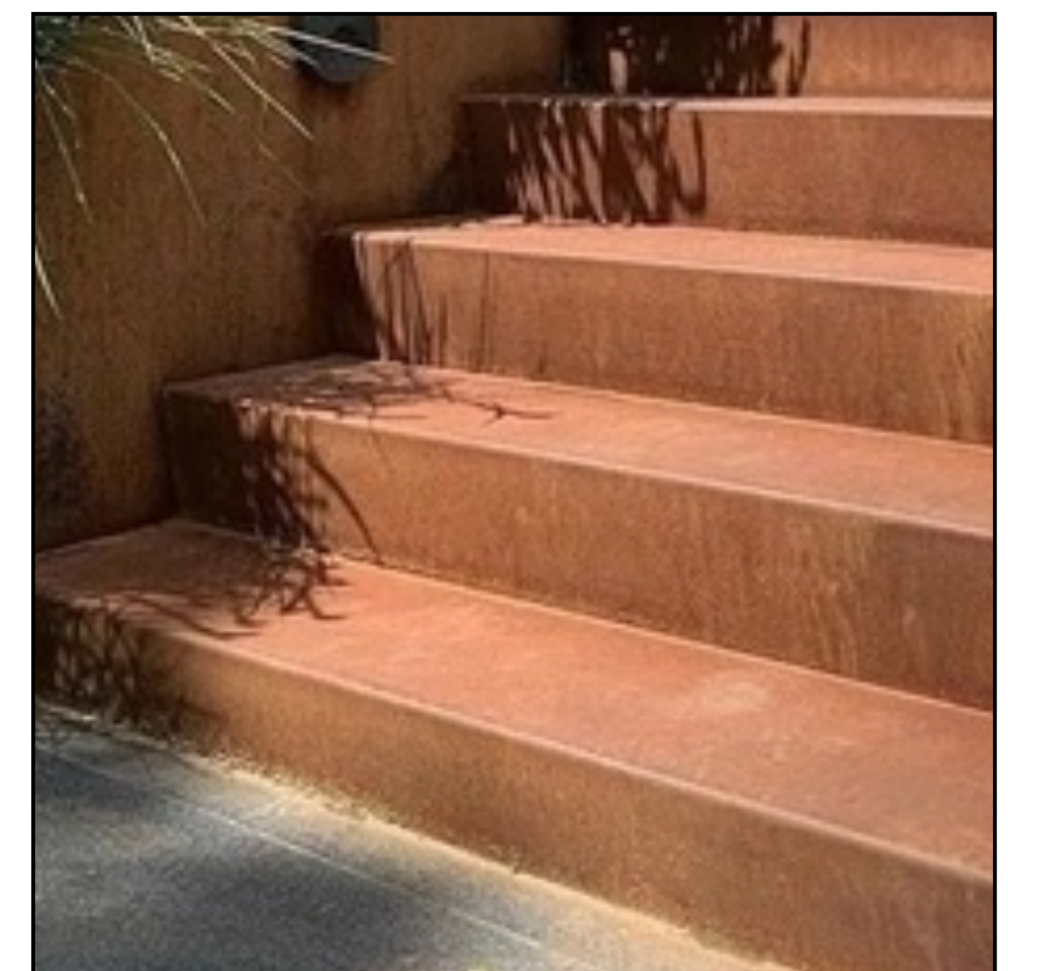
F Corten steel exterior stair
